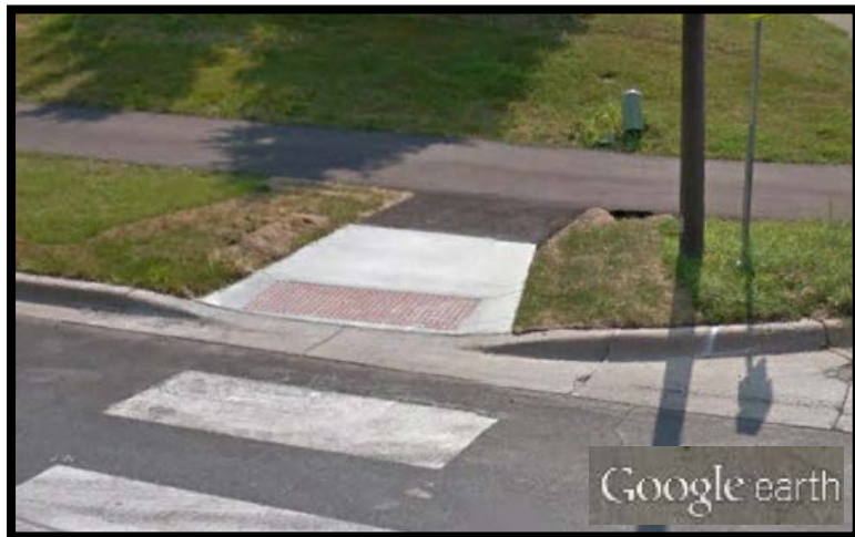
Figure 4.11 Curb Ramp with Landing and Truncated Domes [14] Eagan
