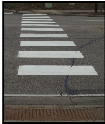
Figure 7.6 High Visibility Continental Crosswalk Markings
