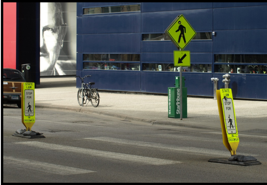
Figure 4.25 Pedestrian Crossing Warning Sign plus In-Road Signs
