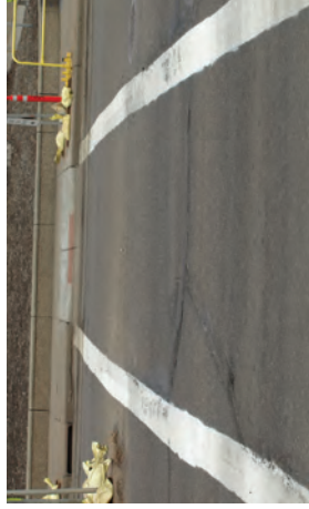
STANDARD/TRANSPOSE CROSSWALK PAVEMENT MARKINGS
