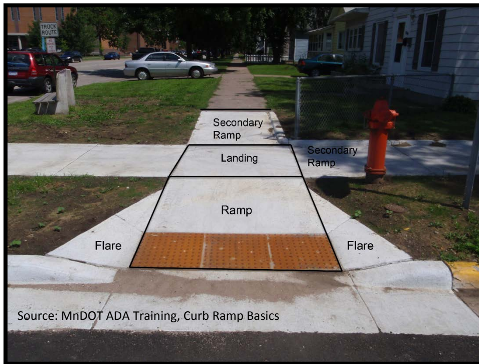
Figure 4.8 Curb Ramp Elements
