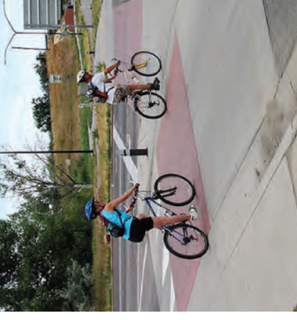
CHANNELIZED TURN LANE WITH RAISED CROSSING
