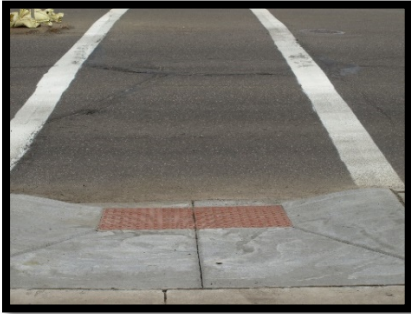
Figure 7.2 Standard Crosswalk Markings
