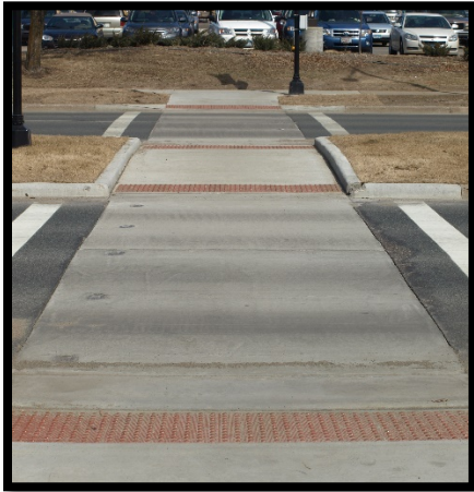
Figure 7.13 Center Median with Refuge Island
