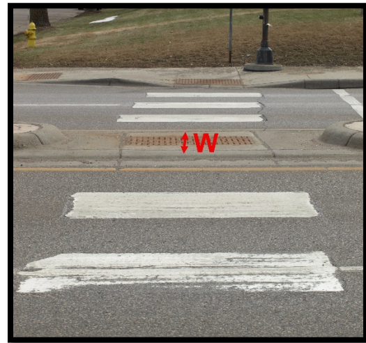
Figure 4.5 Median Width (2 of 2) Not ADA Compliant
