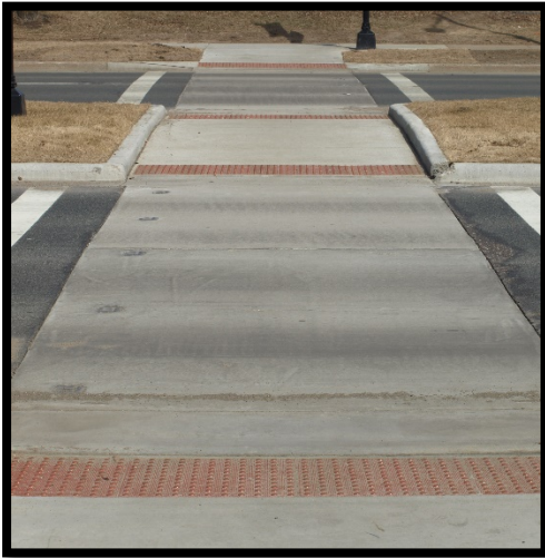
Figure 7.7 Center Median with Refuge Island
