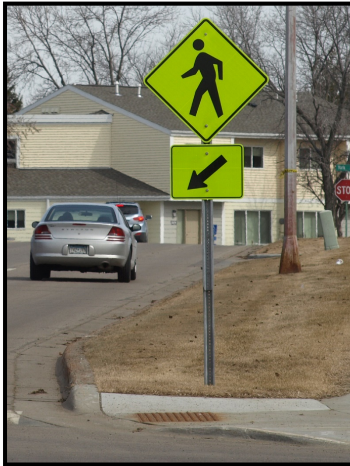
Figure 4.24 Pedestrian Crossing Warning Sign (W11-2) Placed at the Crossing Location
