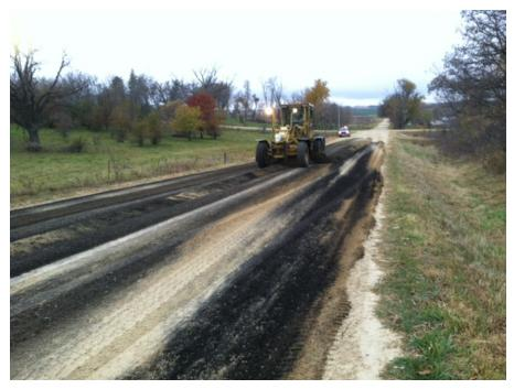
Figure 6 Goodhue CR 6 placing shingles on Cl 6 limestone
