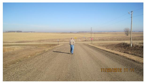
Figure 4 Jackson Co. Looking toward CR 81 on 750th Str. 1 part shingle to 1 part gravel blend
