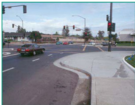
Curb Extensions, City of Minneapolis Source: City of Minneapolis Pedestrian Master Plan
