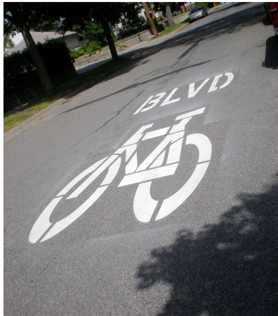
Example pavement marking designating a bicycle boulevard
