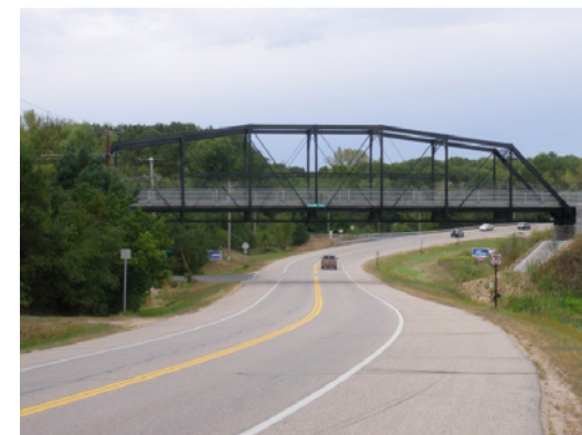
Thinking Outside the Box – This trail overpass on the Gateway Trail in Washington County is a recycled highway bridge from Koochiching County!
