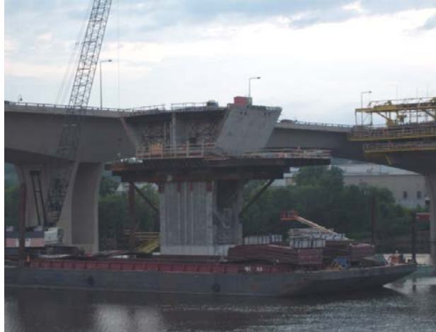
Figure 1.6: Wakota Bridge under construction.
