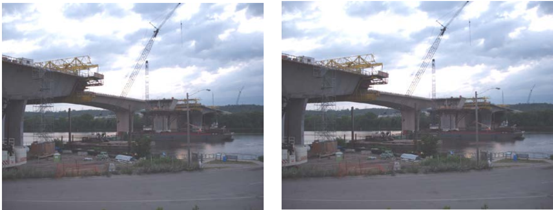
Figure 1.7: Cast in place cantilever construction progress.
