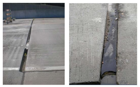
Figure 6: Failures of E8 expansion joints.
