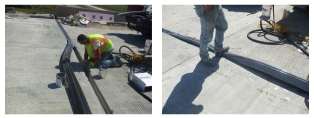
Figure 28: Installation of D.S. Brown JP series compression seal.
