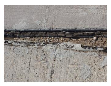
Figure 27: Failed JP-series compression gland.
