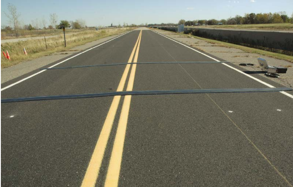
Figure 10: Two-lane single-strip weigh-pads installed on the MnRoad test site
