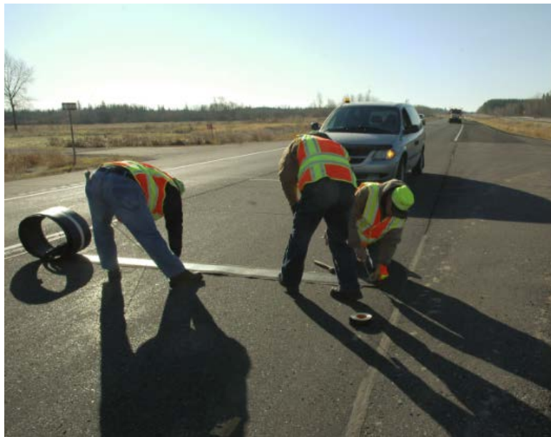
Figure 34: Weigh-pad installation at Cotton, Minnesota, TH-53
