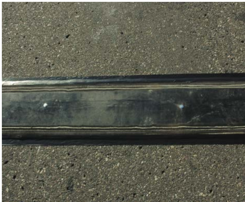
Figure 35: Sleeve anchor screws are fastened in 2 ft. spacing
