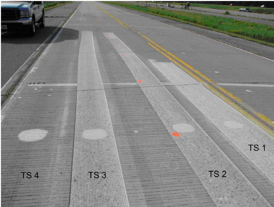
*Figure 2.6. Grinding configurations in Cell 37, looking westbound.*
