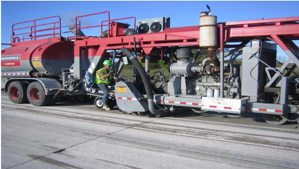
*Figure 4.9. The ultimate diamond grinding process.*
