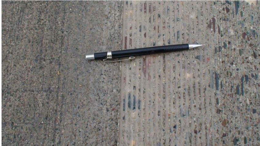
*Figure 4.3. Conventional grind configuration (0.125X 0.125x.0.120).*
