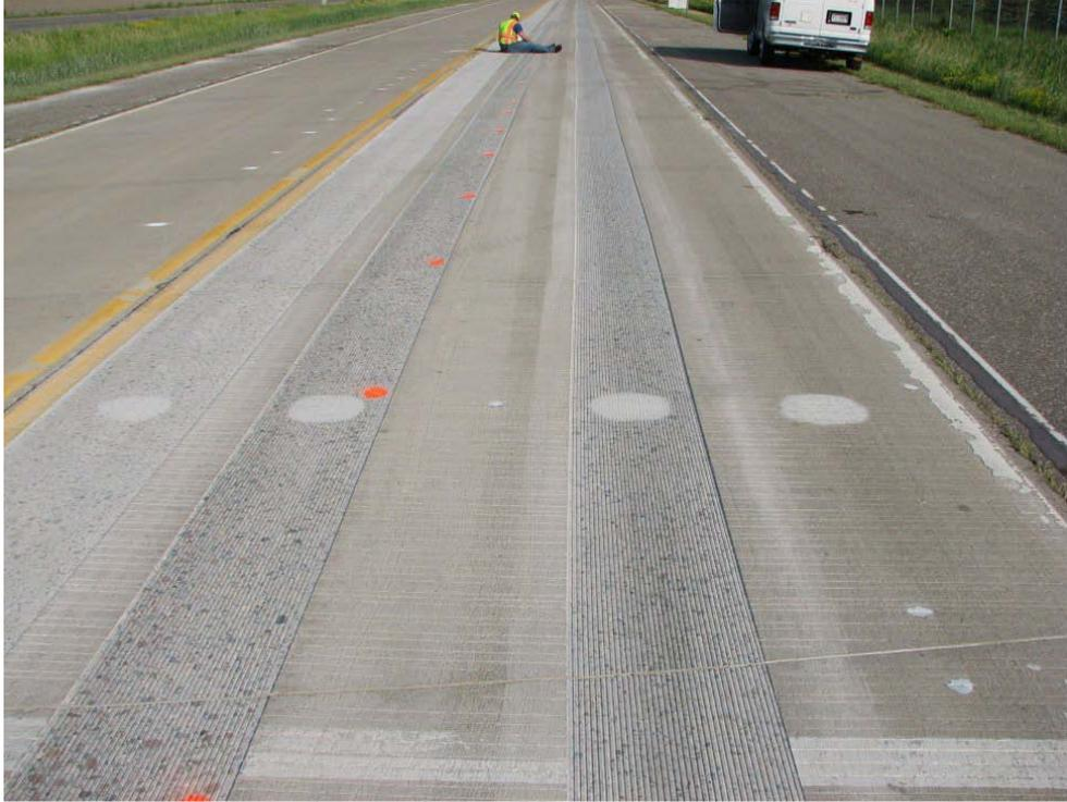
*Figure 2.8. A panoramic view of the texture strips looking west on Cell 37.*
