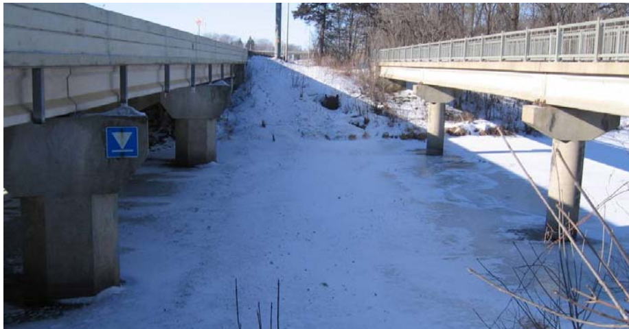
Figure 7.6: Bridge 6868/6869 - upstream pier profiles looking west
