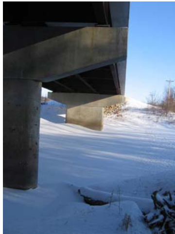
Figure 7.15: Bridge 07038 - upstream pier profiles
