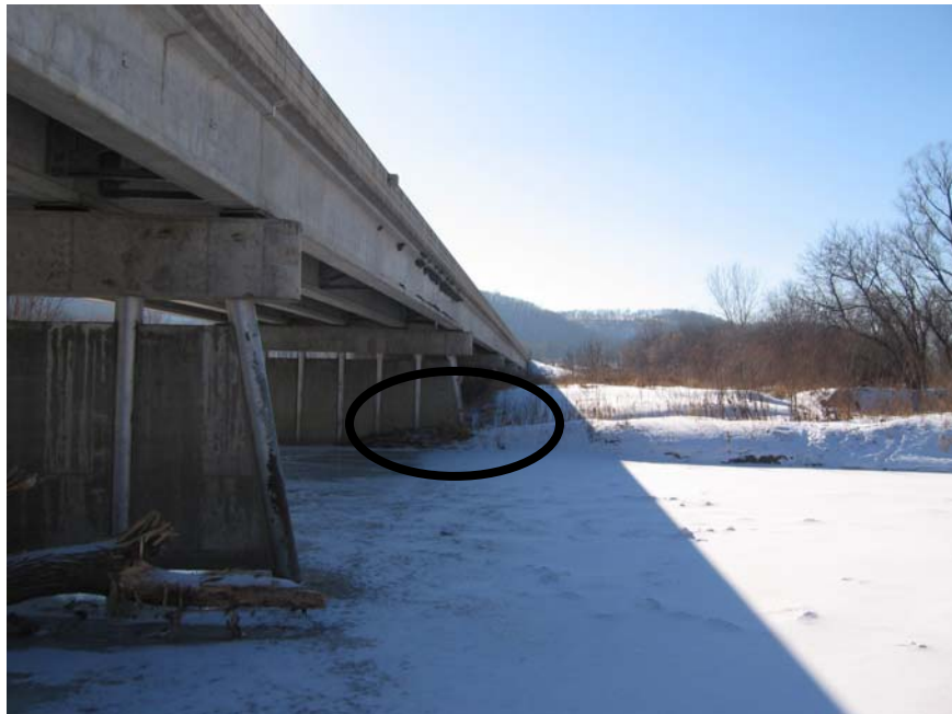
Figure 4.4: Point bar after deposition around pier 4 - looking west (January 2009)
