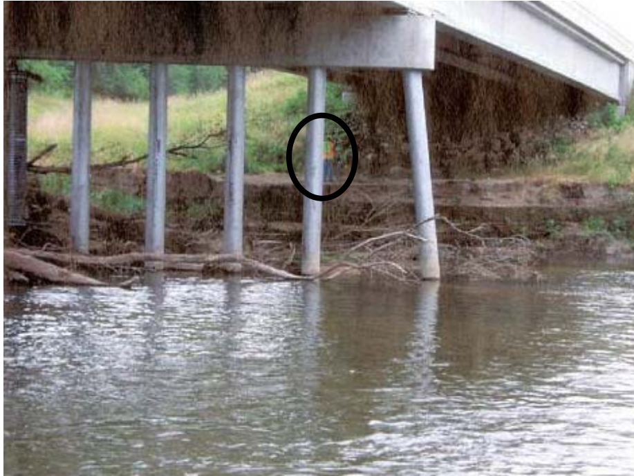
Figure 4.5: Bank erosion due to channel migration - looking east (note scale of person)
