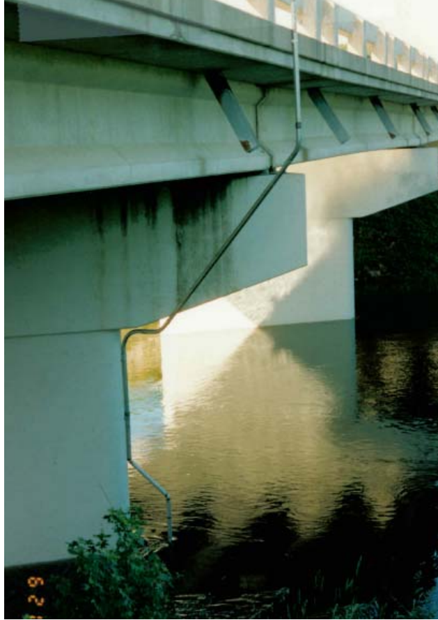
Figure 4.2: Installed manual sliding collar on Bridge 74004
