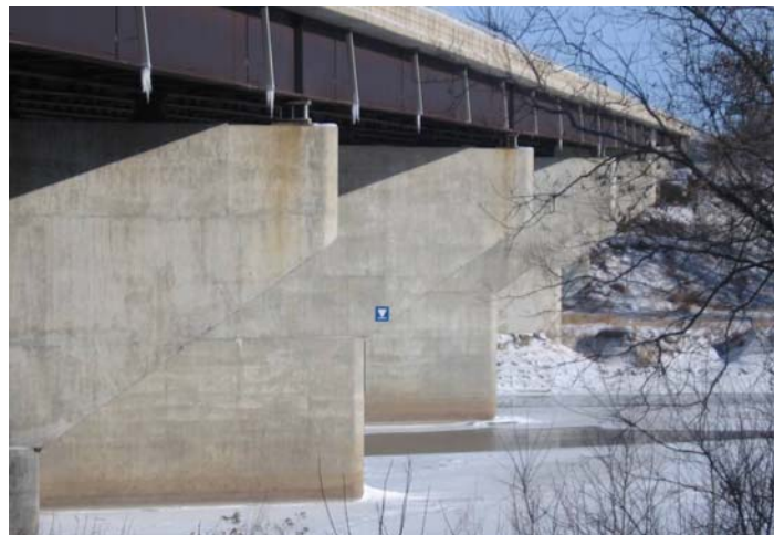
Figure 7.11: Bridge 07011 - upstream profiles of piers 3 through 6
