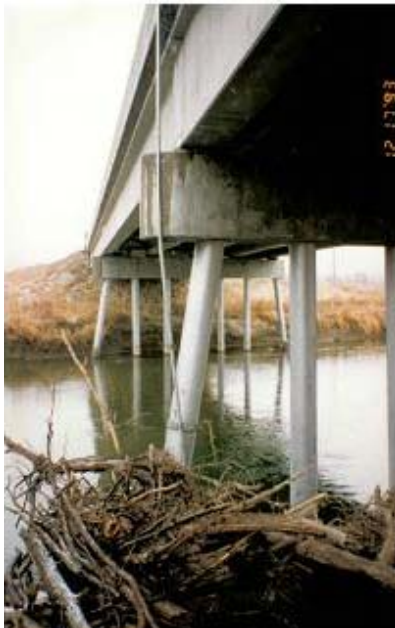
Figure 4.7: Installed manual sliding collar monitor on Bridge 23015 with debris damage
