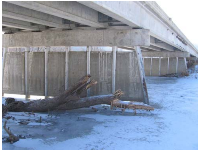
Figure 7.21: Bridge 23015 - upstream pier profiles and debris
