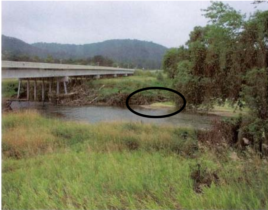
Figure 4.3: Point bar before deposition around pier 4 - looking west (unknown date)
