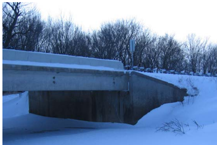
Figure 7.2: Bridge 6468 - upstream left abutment
