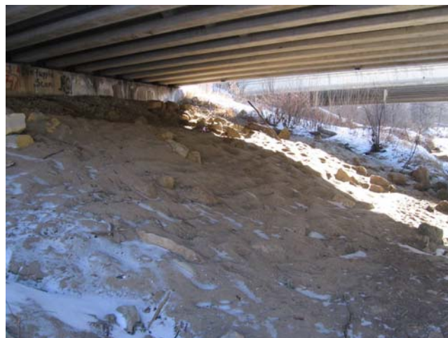
Figure 7.7: Bridge 6868/6869 - sand covered riprap on east abutment
