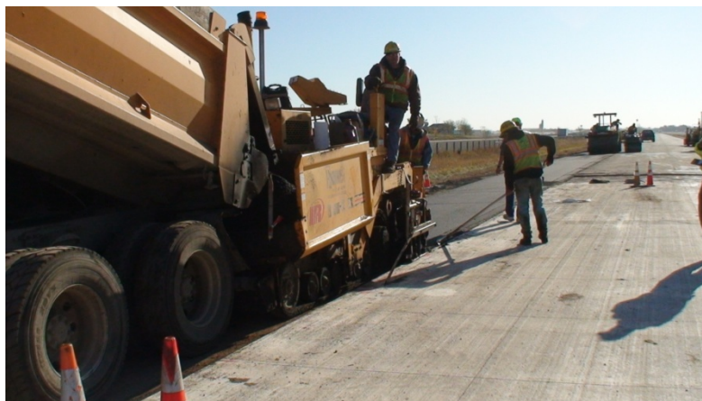
Figure 5.6. MnROAD MWSS Shoulder Construction
