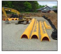
Underground Storage & Infiltration -Source: Minnesota Stormwater Manual
