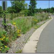
Infiltration Trench - Source: Minnesota Stormwater Manual
