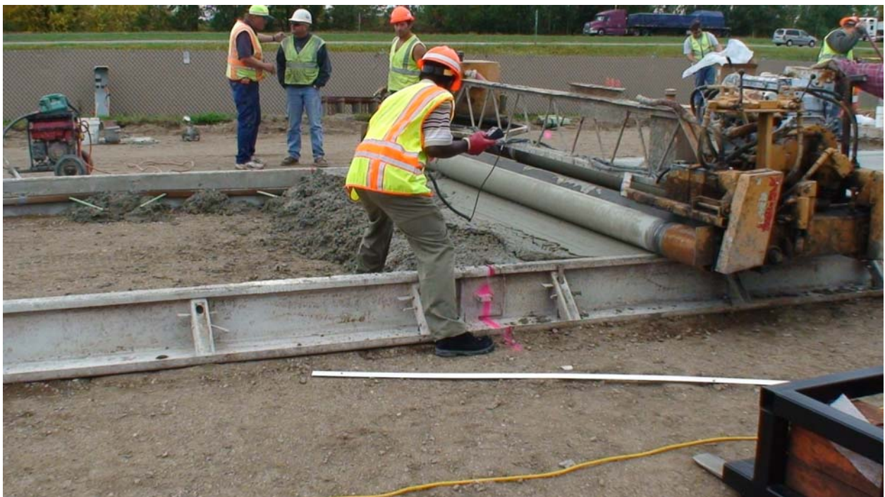
Figure E2. McCleary screed used to compact the concrete.
