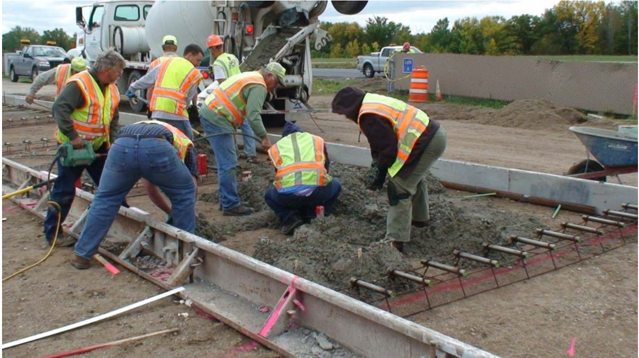
Figure E1. Placement of concrete around sensors.
