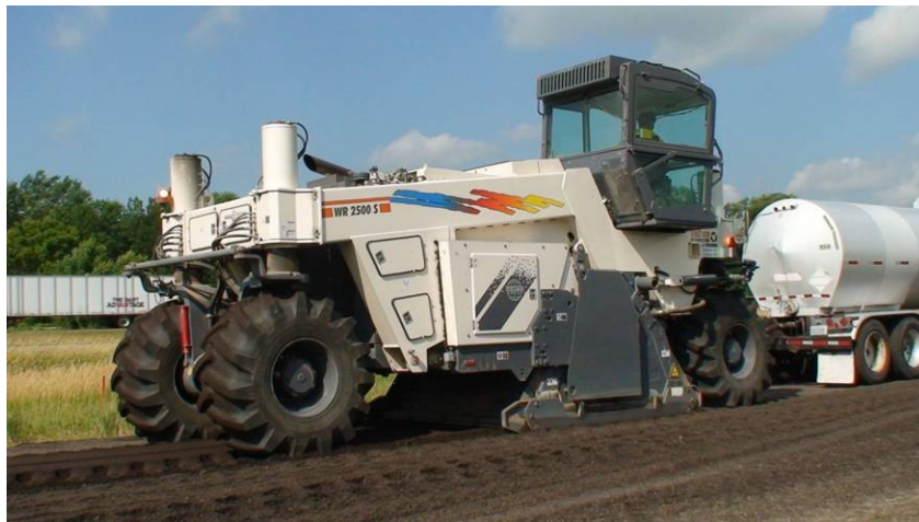
Figure 36. Asphalt Emulsion Application to Reclaimed Material
