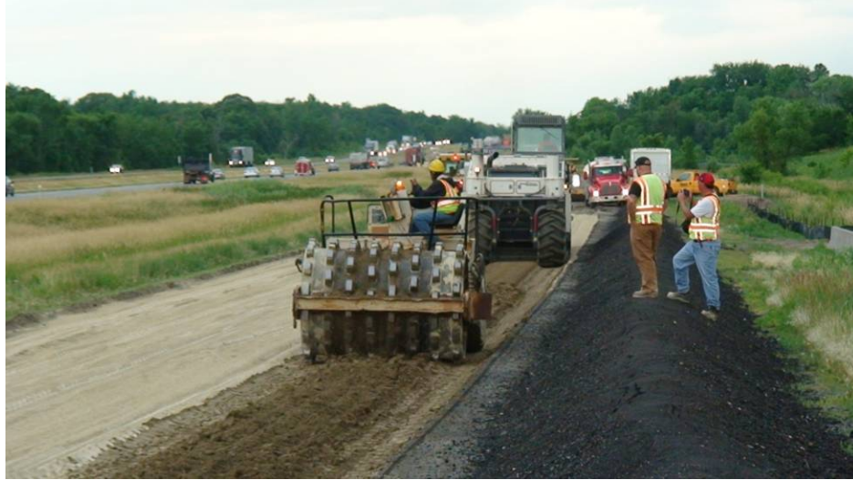
Figure 35. Reclaiming and Compacting Cell 2
