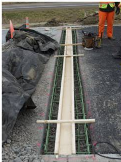
Figure 26. Transverse Drains in Cells 85-89
