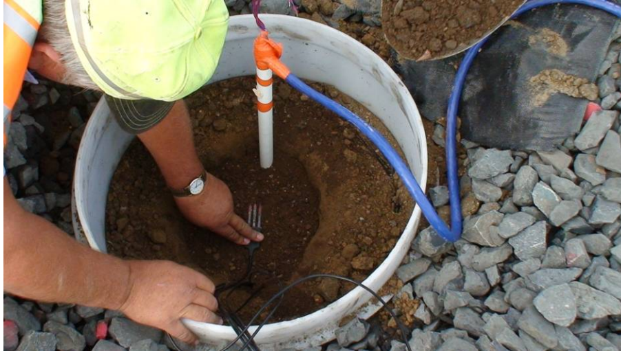
Figure 37. Installation of Moisture and Temperature Gauges in Cell 23
