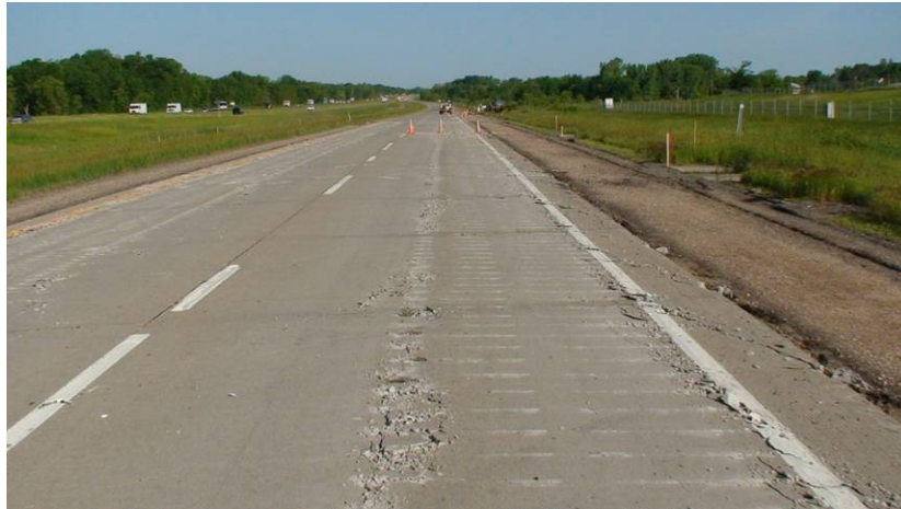
Figure 33. Concrete after Breakup by Road Warrior
