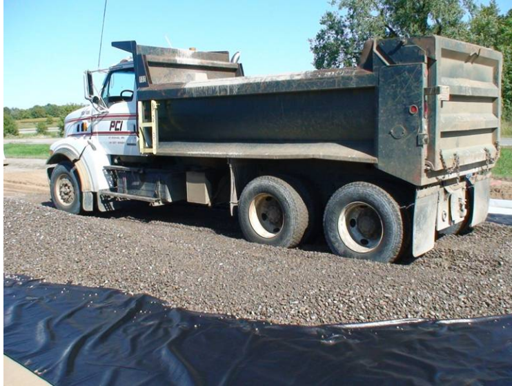
Figure 38. Geotextile and CA-15 Base in Cells 85-89
