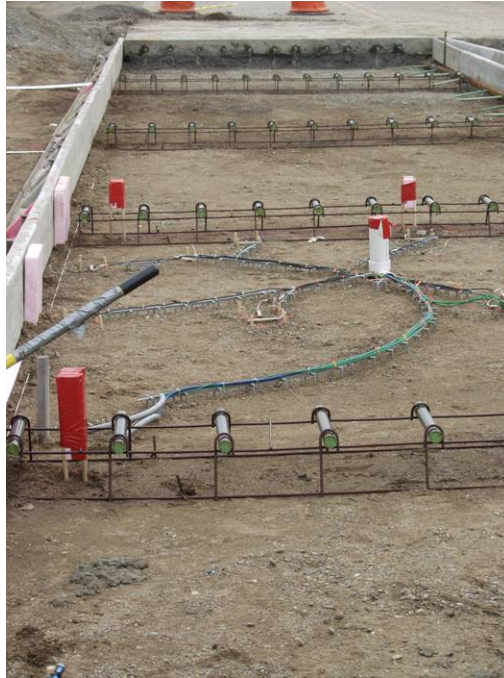
Figure 19. Cell 53 Sensor and Dowel Bar Layout
