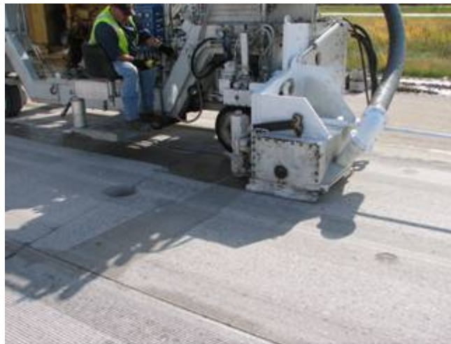
Figure 14. Cell 9 Diamond Grinding
