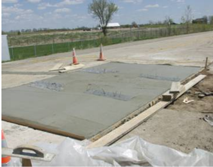
Figure 27. Sensor Retrofits Installed on Cell 39
