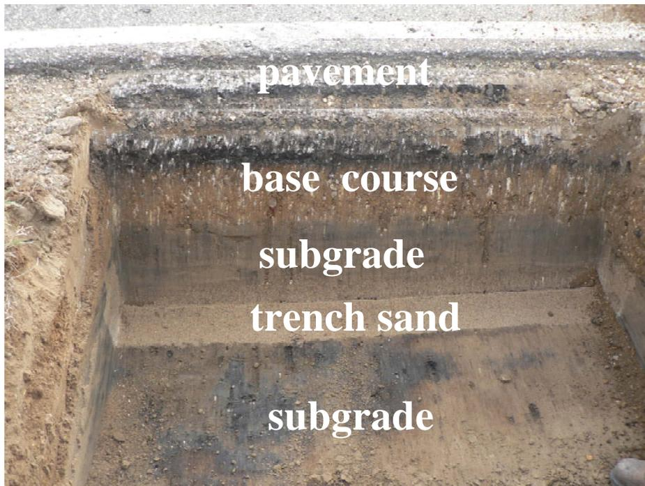
**Figure 7.2 Illustration showing the excavated pit down to the level just above the edgedrain elevation**
