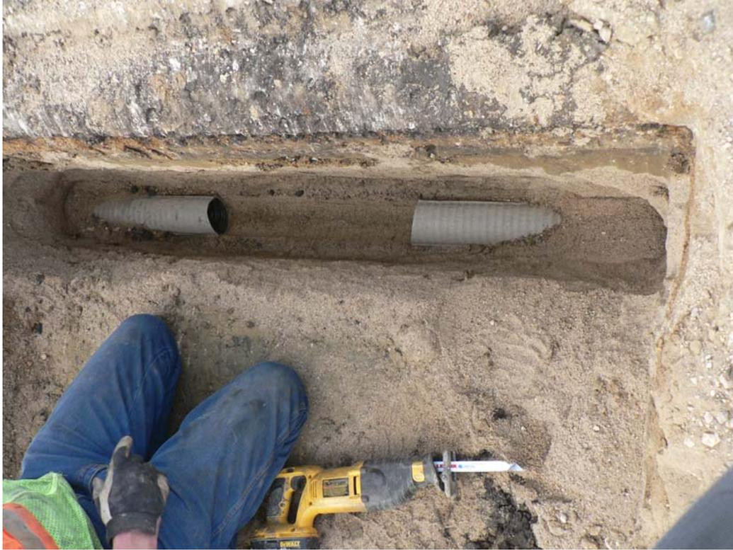
**Figure 7.5 Edgeline with tile sample removed**
