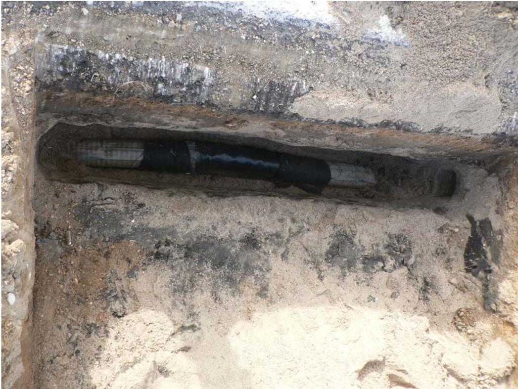
**Figure 7.6 The edgeline with the splice in place**
