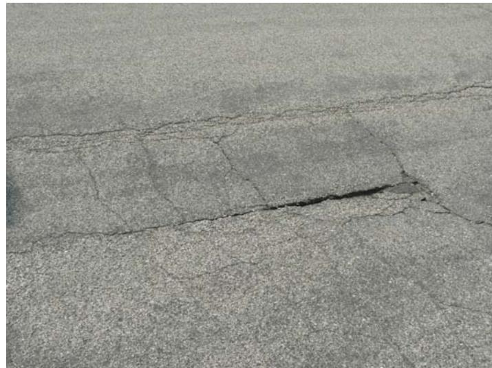
**Figure 8.5 Closeup view of cracking on Pleasant Street**
