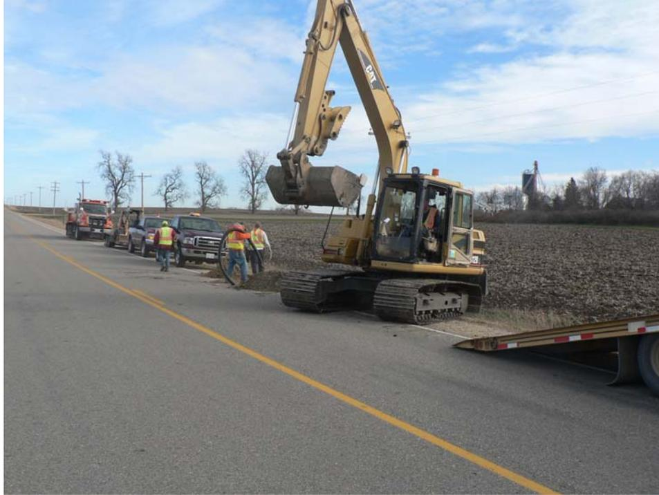
**Figure 7.1 Illustration of the tracked backhoe machine used to excavate through the unpaved shoulder to access the edgedrain tile on Nobles County CR 32 and CR 35**
