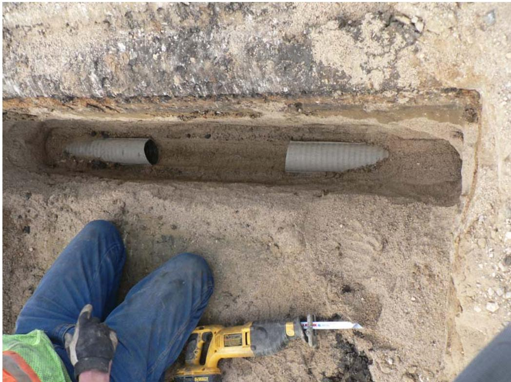
**Figure 7.5** Edgedrain with tile sample removed
