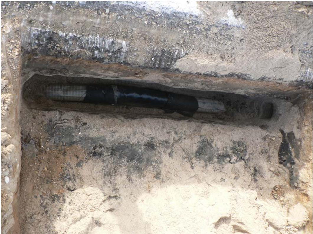
**Figure 7.6** The edgedrain with the splice in place
