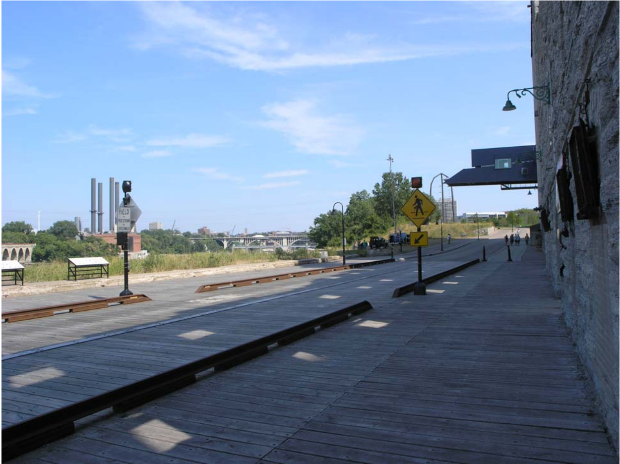
Figure B-16. Site 16 (see table above). Pedestrian-actuated warning crosswalk in Minneapolis across West River Parkway, looking east.
