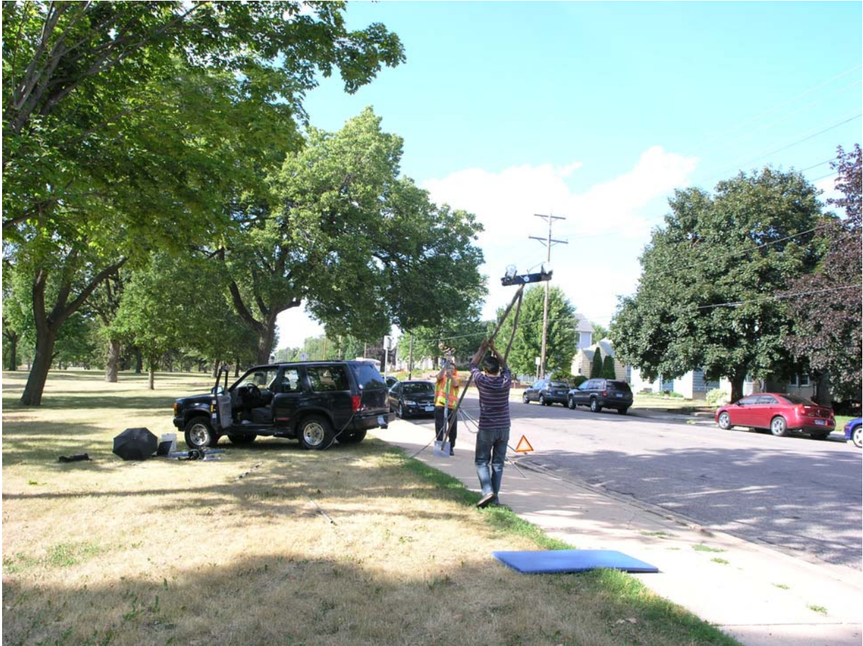
Figure E-4. Erecting camera boom after base of boom has been inserted into hitch assembly (photograph taken at different site from the site portrayed in preceding and following photographs).
