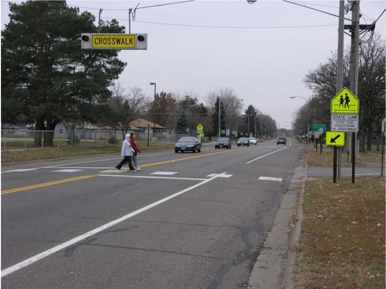
Figure B-12. Site 12 (see table above). Continuously active warning crosswalk in Coon Rapids across Northdale Blvd., looking east.
