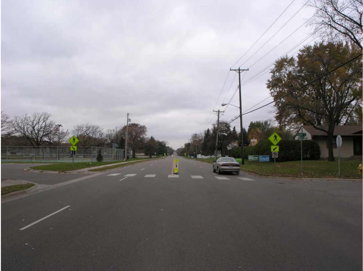
Figure B-1. Site 1 (see table above). Passive warning crosswalk in Roseville across County Road C at Galtier St., looking west.
