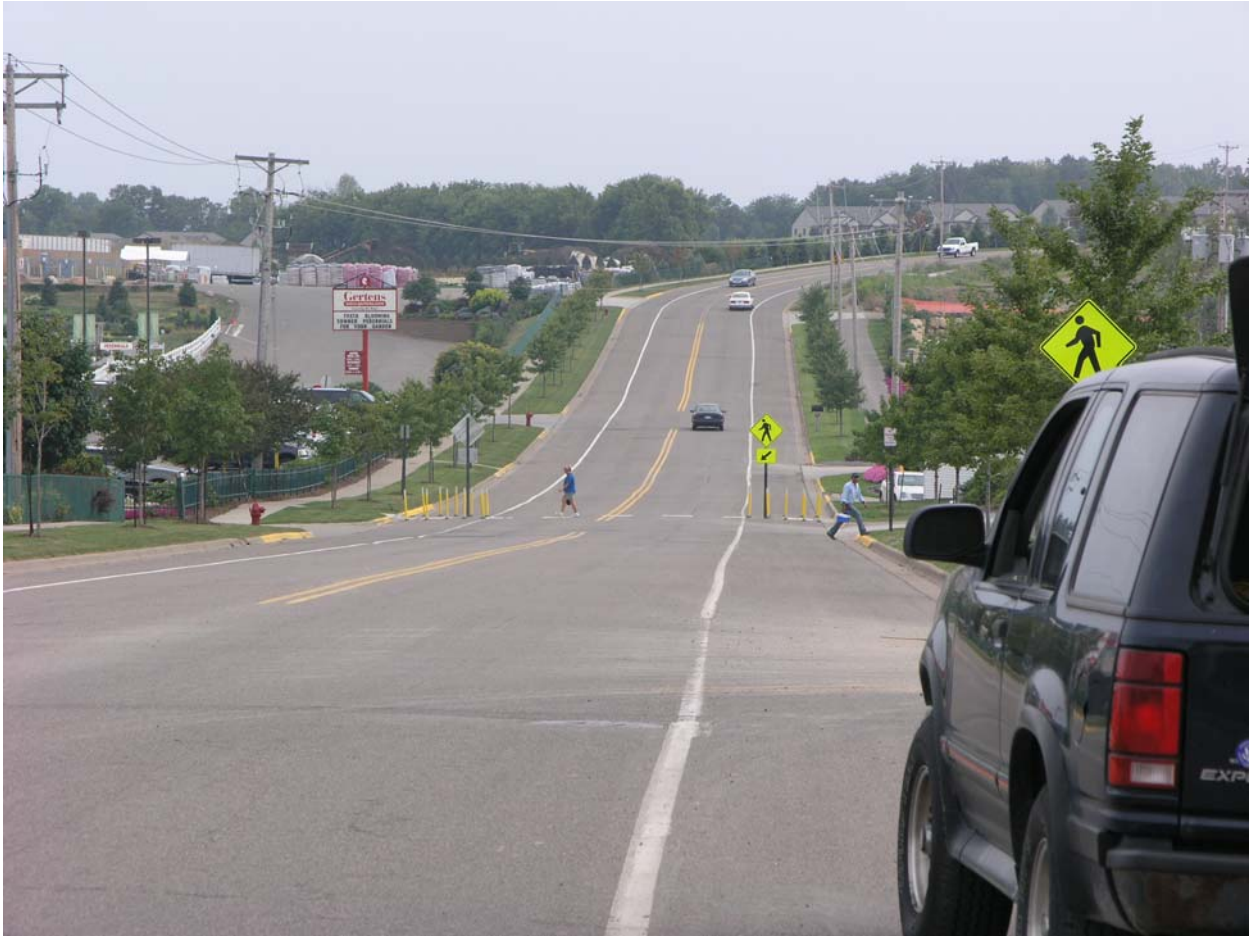
Figure B-5. Site 5 (see table above). Passive warning crosswalk in Inver Grove Heights across Blaine Ave., looking south.
