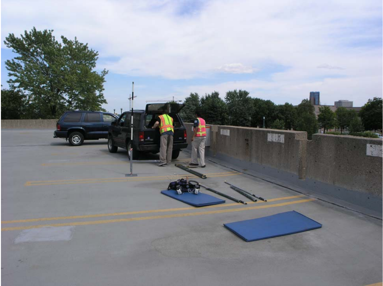
Figure E-1. Laying out camera boom components. The black and white banded pole is the calibration stick inserted (temporarily) in the hitch assembly.
