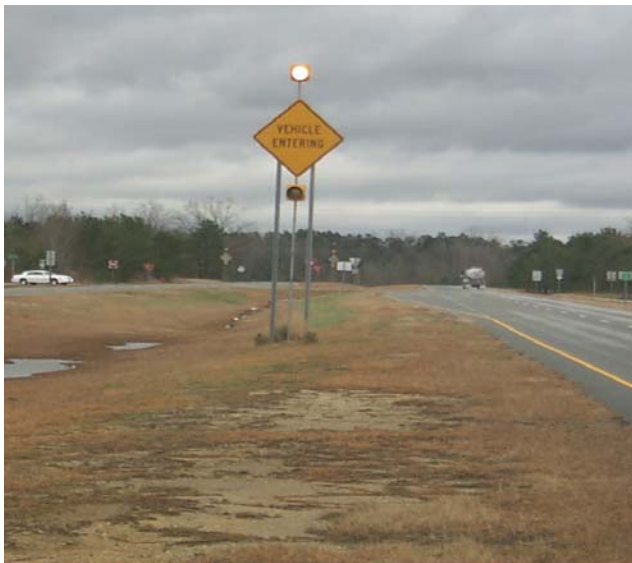
FIGURE 2-3 Dynamic Mainline Warning Flashers at a North Carolina Intersection Used to Alert Mainline Drivers
