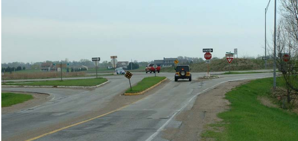
FIGURE 2-2 Splitter Island at an Iowa Intersection Used to Increase Approach Visibility
