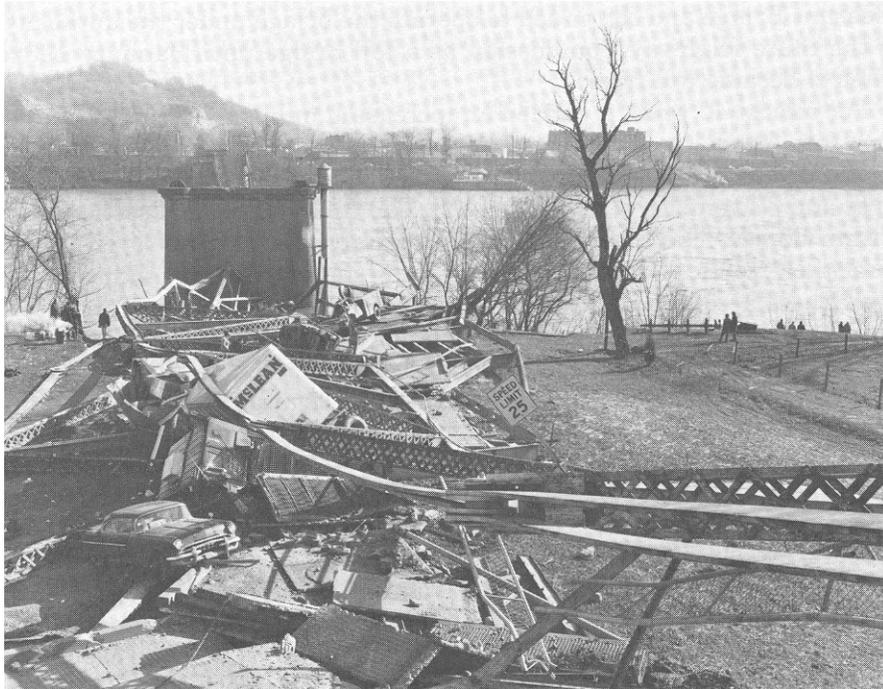
**Figure 3.3** Collapse of Point Pleasant (Silver Bridge) (Fisher 1984)
