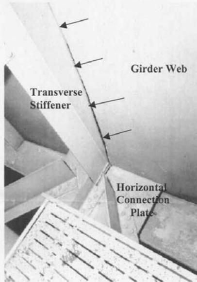
0 *Transverse Groove Welds* – Groove welds to web of girders. Usually occur at the end of horizontal stiffeners or the end of haunch inserts.
