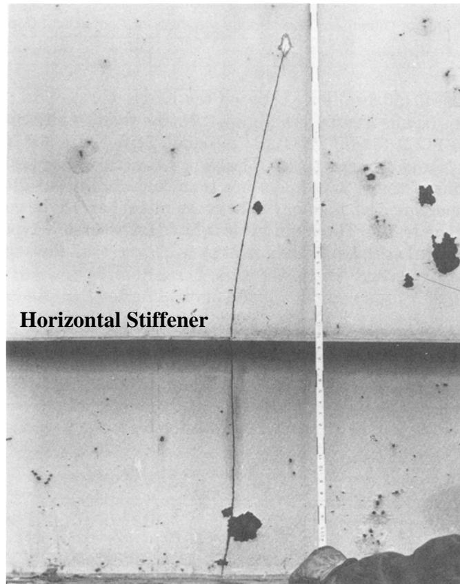
**Figure 2.12** Crack in girder web of Quinnipiac River Bridge (Adapted from Fisher 1984)
