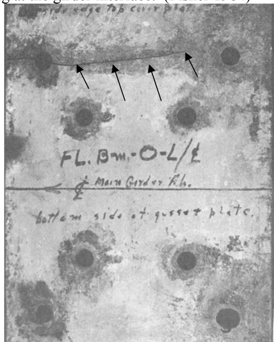
**Figure 2.15** Crack through tie plate of Allegheny River Bridge (Adapted from Fisher 1984)
