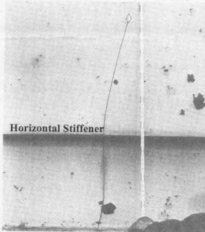
7 *Web penetrations* – When a member passes through the web of another. Cracking is more common when backing bars are left in place. These details are common in pier caps.
