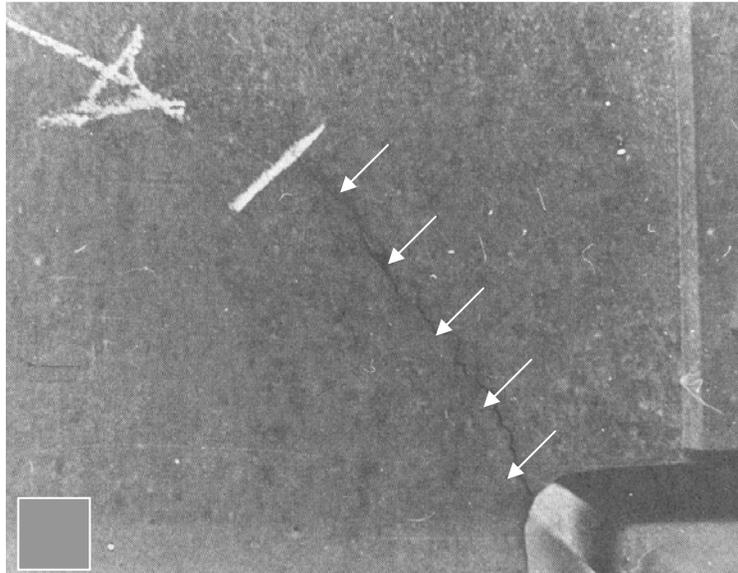
**Figure 2.7** Crack originating from the coped stringer of Hwy 51.5 Bridge (Adapted from Fisher 1984)
