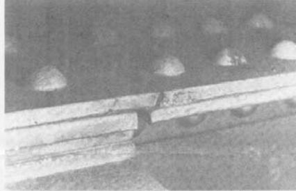
4 *Web Connection Plates* – horizontal plates welded to the girder web. Cracks usually occur when plate intersects a transverse stiffener.
