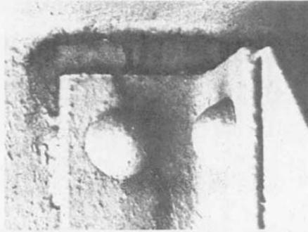
6 *Cantilever floor-beam brackets* – These plates are laid horizontally and usually bolted or riveted to the girders. They are also connected to the top of short beams that extend out from the bridge to increase bridge width. Cracking can occur around tack welds, bolts, rivets, or across the plate as shown.
