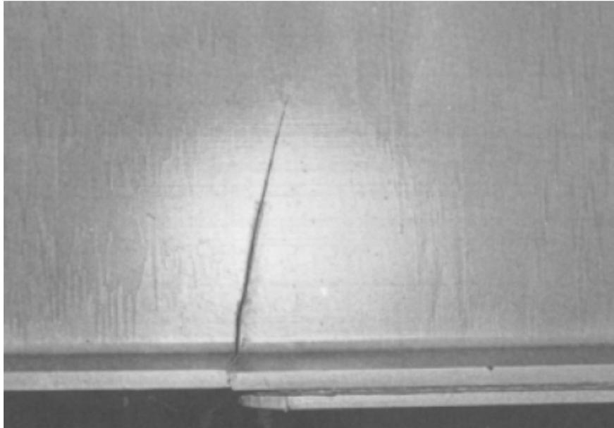
**Figure 2.9** Crack at end of cover plate of Yellow Mill Pond Bridge propagating into web (Fisher 1984)
