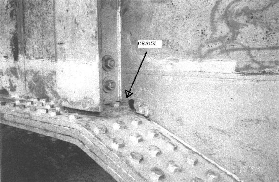
**Figure 5.4** Haunch insert cracking (close-up) - Lexington Avenue Bridge (Wilson, October 2006)
