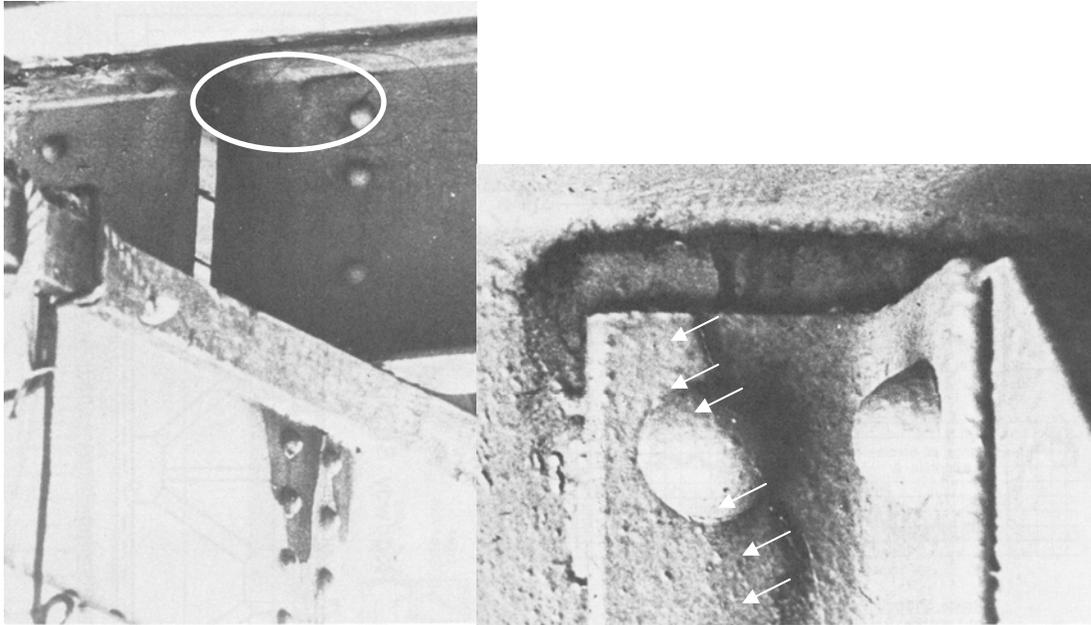
**Figure 2.11** Stringer web cracks above bracket at roadway relief joint of the Walt Whitman Suspension Bridge
