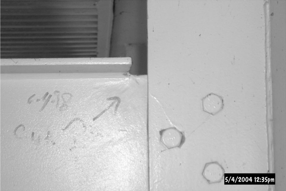
**Figure 8.6** Insufficient cope radius (Bridge # 9320)
