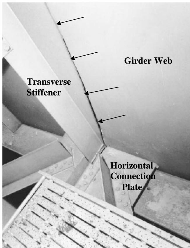
**Figure 2.10** Cracked girder of Lafayette Street Bridge (Adapted from Fisher 1984)
