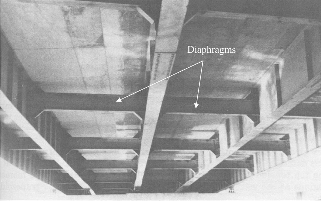
**Figure 2.3** Diaphragms and transverse stiffeners on steel girder bridge (Fisher 1984)
