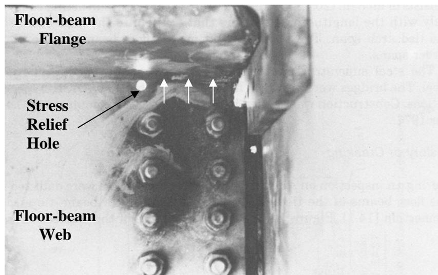
Figure 2.17 Cracking of floor-beam and floor-beam connection plate (Adapted from Fisher 1984)
