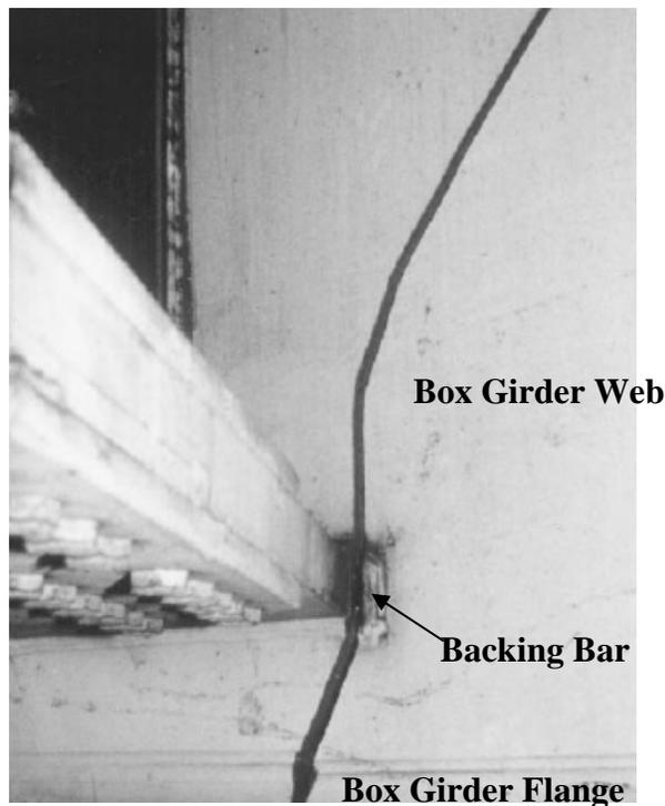
**Figure 2.14** Crack through webs and flange of Dan Ryan Rapid Transit Structure (Adapted from Fisher 1984)
