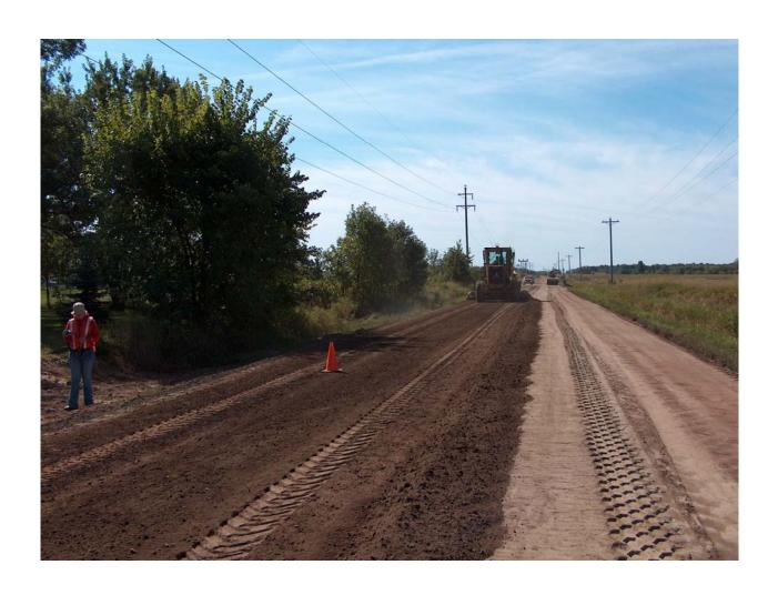
Fig A10. Compaction and grading of S-RSG surface.
