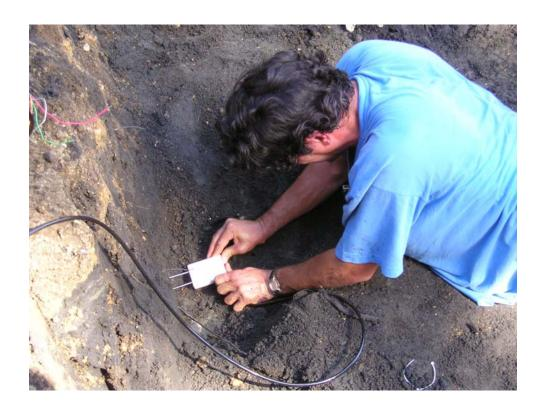
Fig. B3. Installing water content reflectometer in subgrade.
