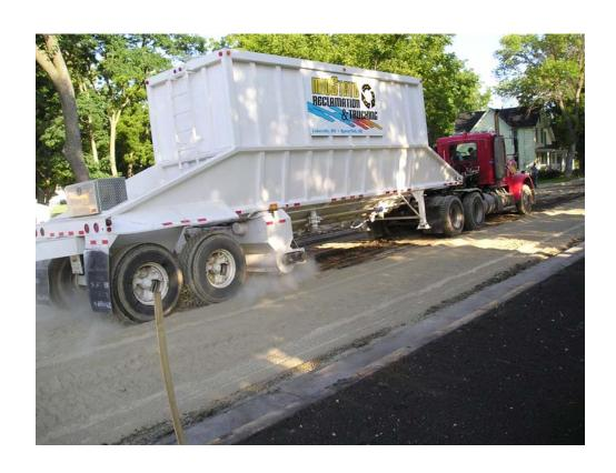
Fig. A2 Lay-down truck placing fly ash on SRPM.
