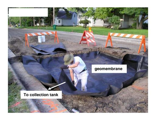
Fig. B1. Installing geomembrane for lysimeter.
