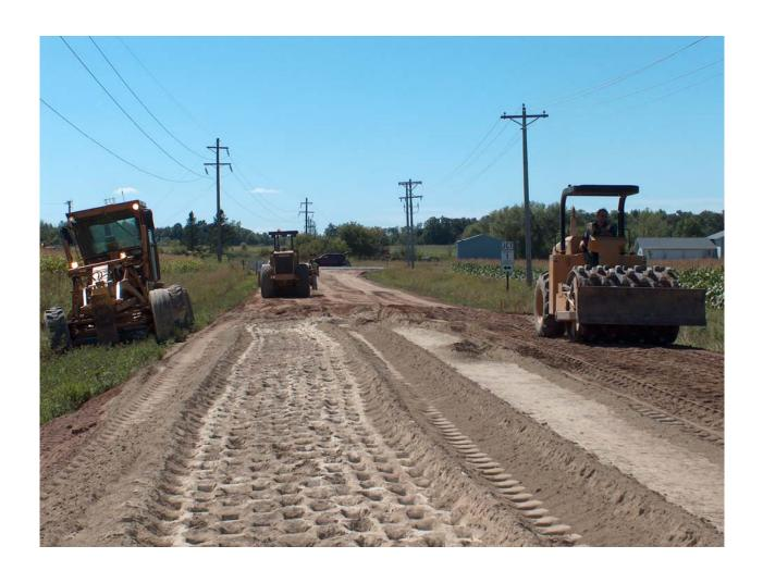
Fig A9. Compaction of fly ash and RSG mix by using sheep foot and roller drum compactors.
