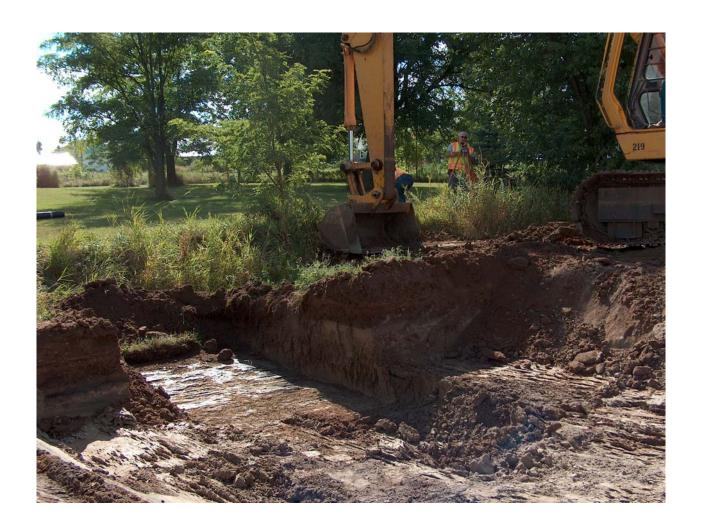
Fig A14. Excavation of lysimeter pit.
