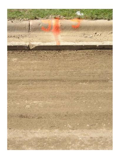
Fig. A4. Surface of SRPM after compaction.
