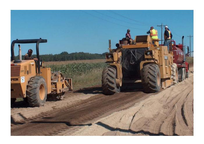
Fig A7. Road-reclaimer blending fly ash and water truck
