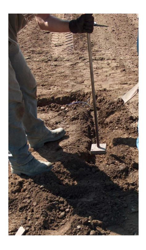
Fig A21. Compcation of sensor trench with a hand compactor in S-RSG
