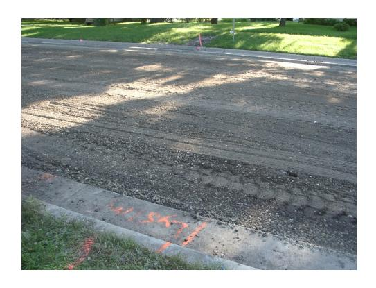
Fig. A1. RPM before placement of fly ash.
