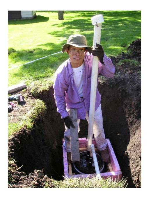
Fig. B2. Installing collection tank for lysimeter.
