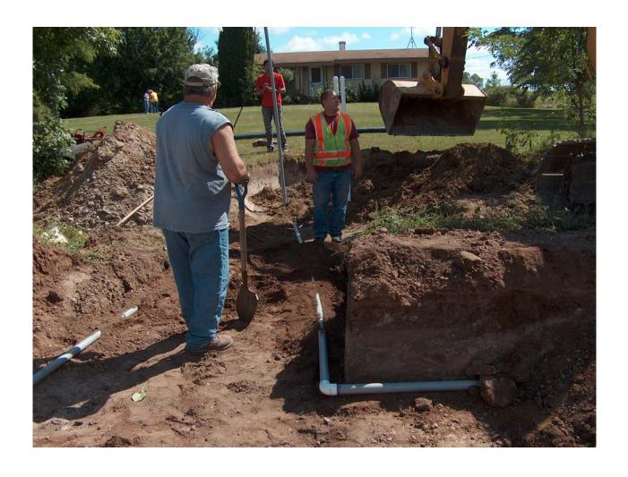
Fig A19. Installation of temperature sensors into subgrade and RSG in lysimeter pit. Sensor 6 is in subgrade and Sensor 5 is in RSG.
