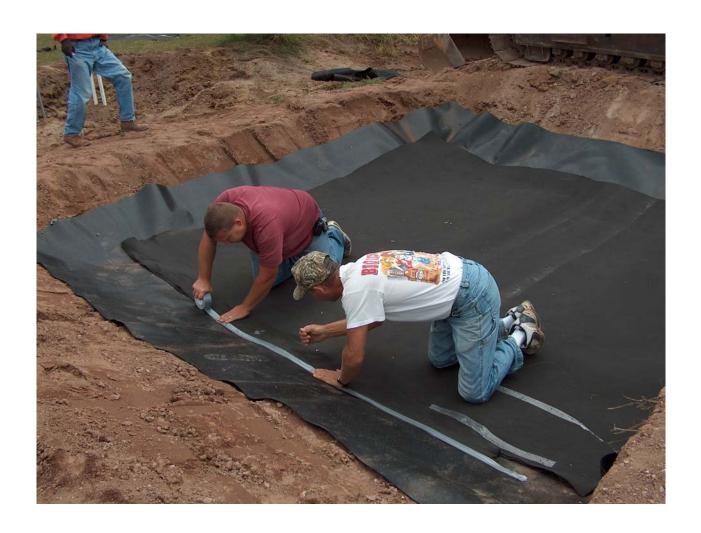
Fig A16. Placement of geomembrane and geotextile.
