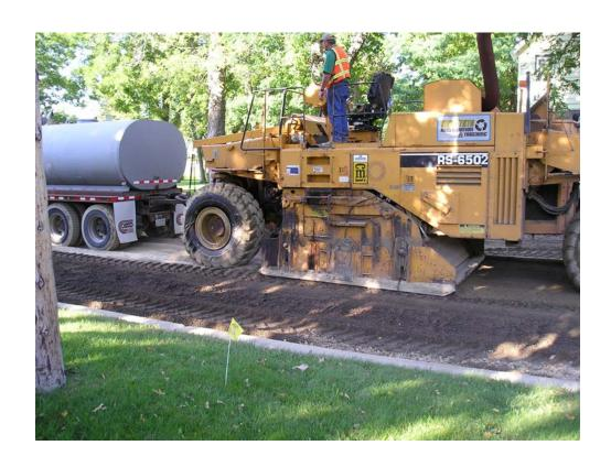
Fig. A3. Water truck and road-reclaimer blending fly ash, water, and RPM.
