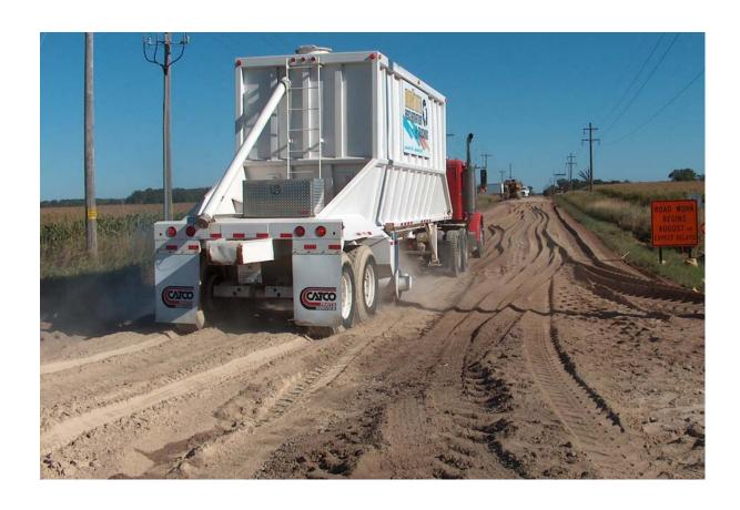
Fig A6. Lay-down truck placing fly ash on RSG
