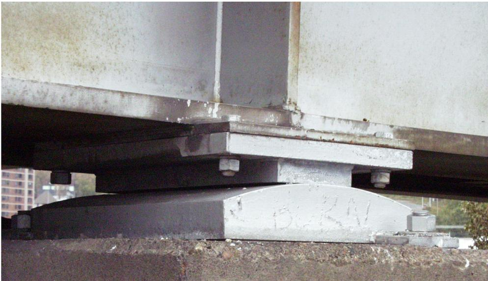
**Figure 3-15: Fixed Bearing at Pier 8**
