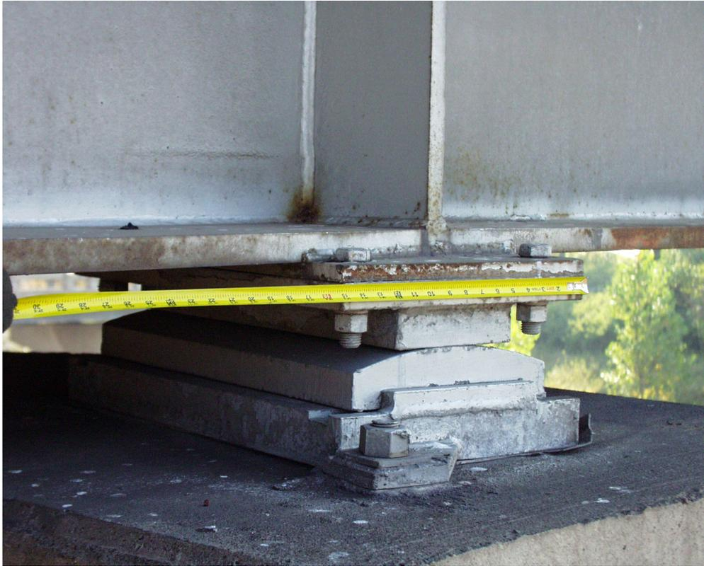
**Figure 3-14: Expansion Bearing at Pier 9**
