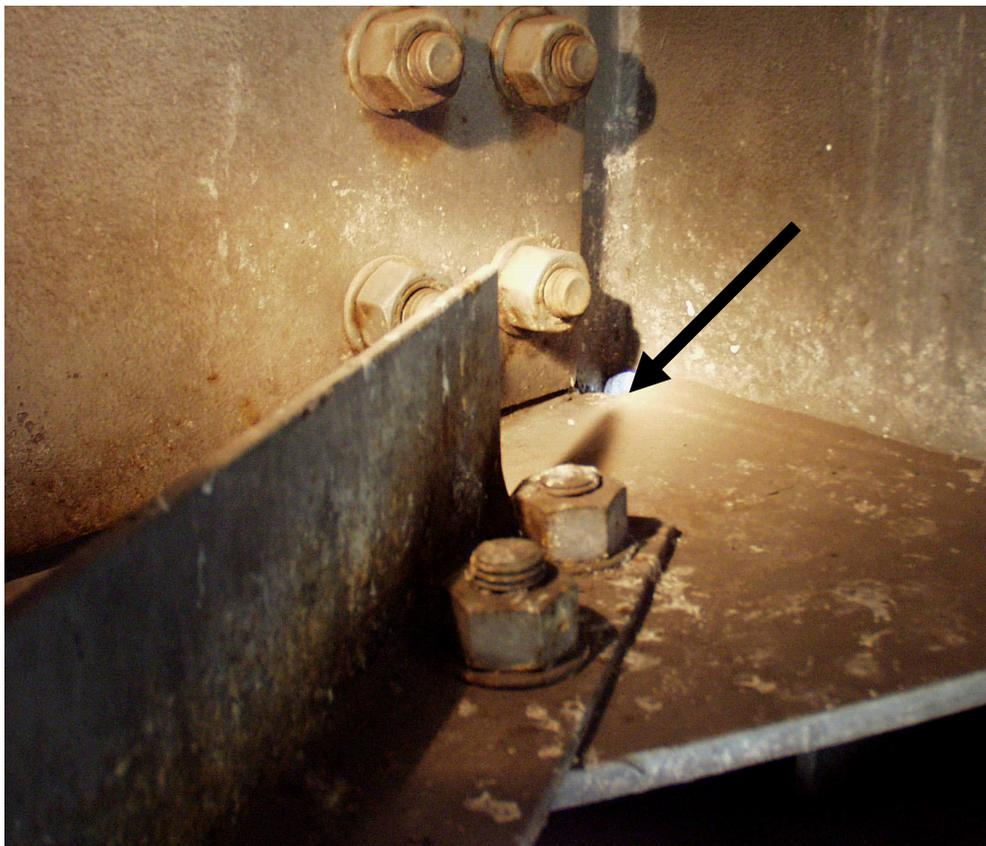
**Figure 3-13: Gusset Plate Retrofit (arrow) from Interior Face**
