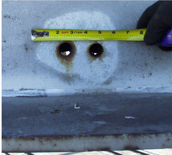
**Figure 3-12: Gusset Plate Retrofit from Exterior Face**
