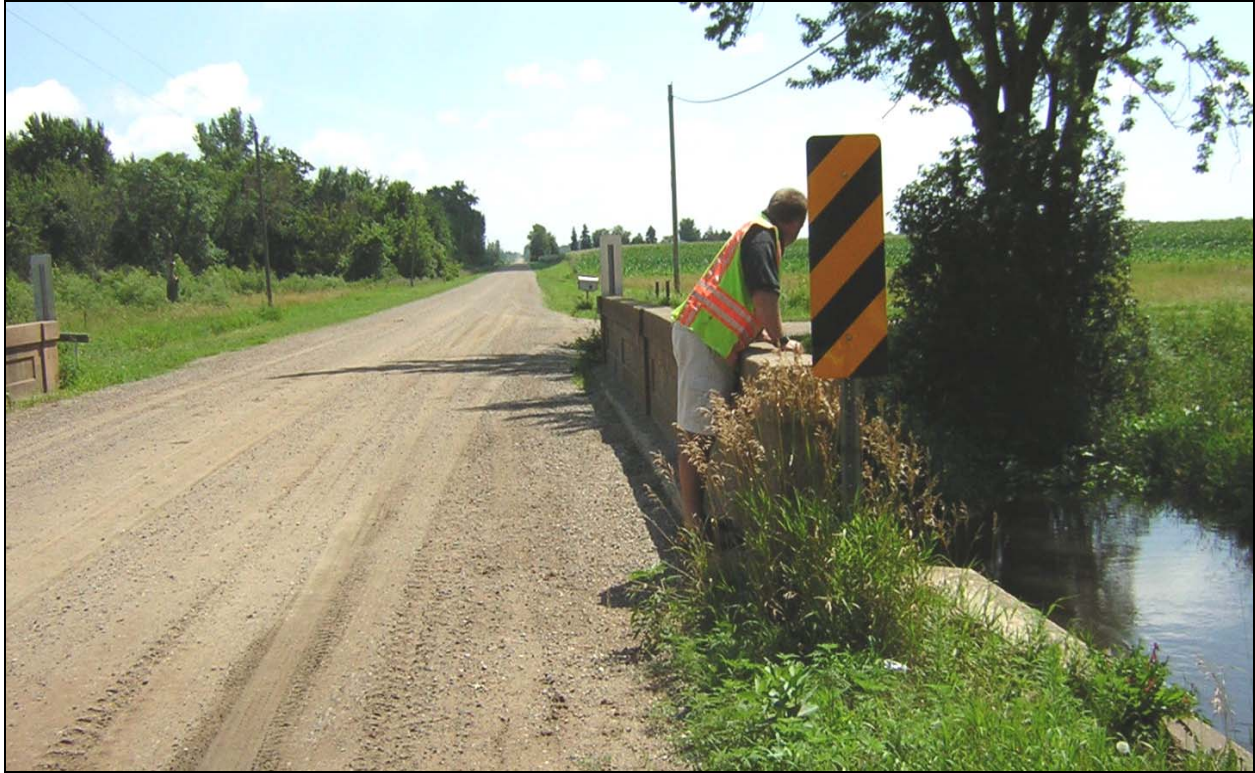
Figure 3.2. CSAH Bridge Without Approach Guardrail
