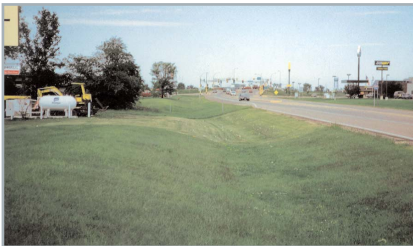
Ditches direct water away from the roadway base.
