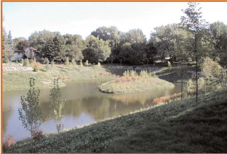
Storm Water Ponds are an excellent way to control and treat runoff.
