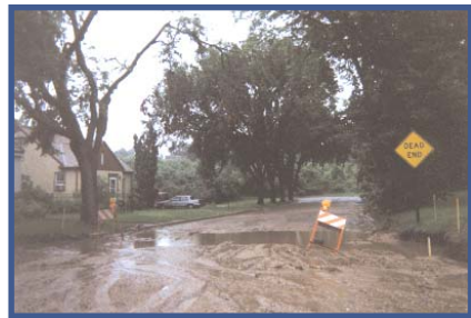
Controlling erosion and sedimentation during construction will prevent muddy roads, like the one shown here.
