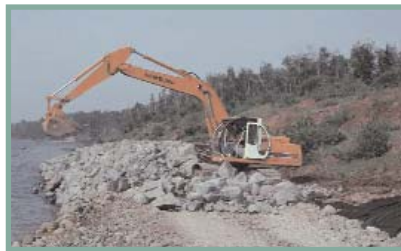
Placing buttress rock and armor stone at toe of slope. Photo courtesy of BWSR.
