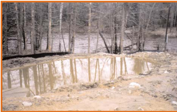
A temporary sediment basin can trap sediment prior to storm water discharge.
