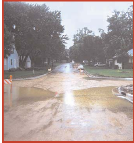
Heavy rains result in erosion during construction.
