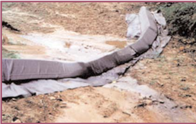
A triangular silt dike slows water and allows sediments to settle. Source: ACF Environmental
