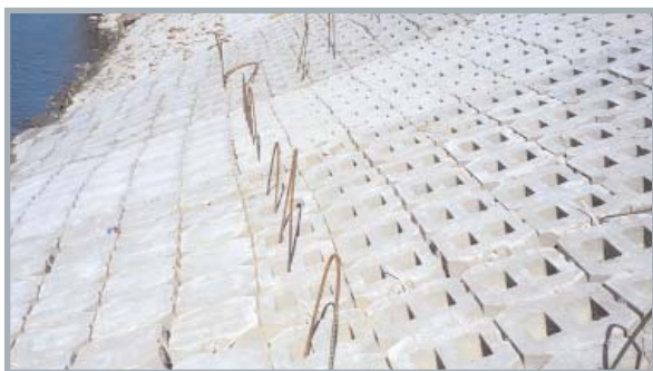
Concrete armor units are useful for stormwater erosion control in high volume and high velocity situations.
