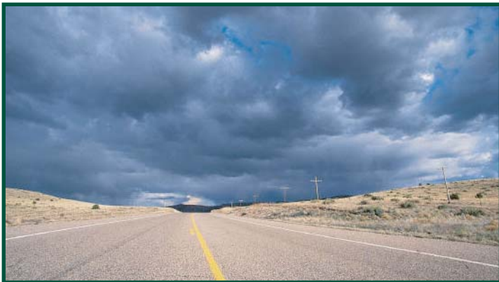
Tracking rainfall events is a important part of inspection.
