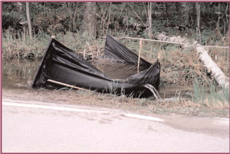
Silt fence as temporary ditch check.
