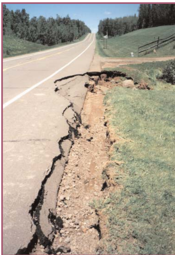
Erosion can cause costly repairs, to the roadside and pavement structure.
