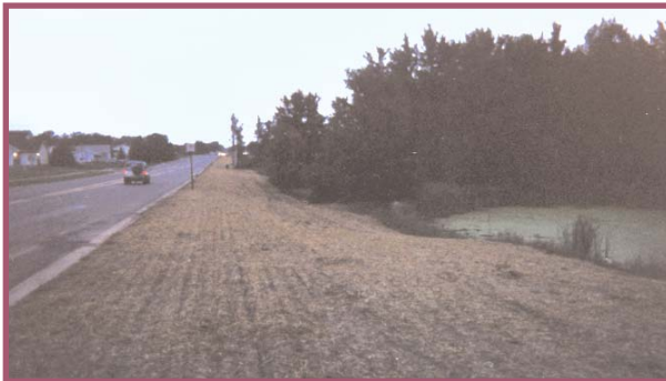
Mulch along road shoulders to stabilize the soil.
