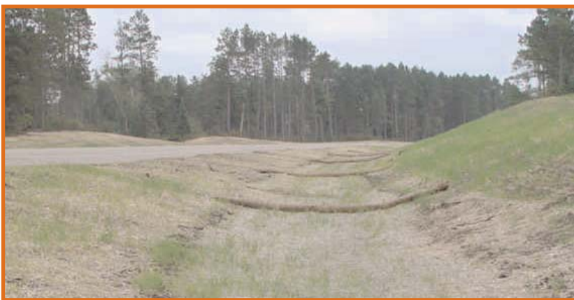
Bioroll application on TH 200 near Bemidji.
