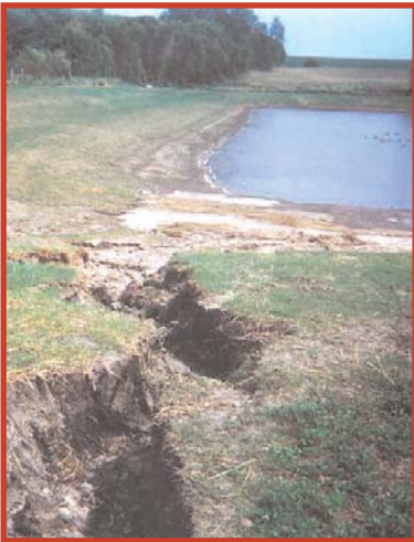
Gully erosion results when small erosion problems are not corrected in time.
