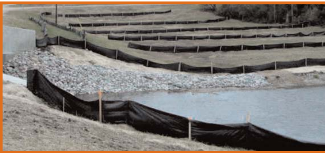
Many tiers of silt fence can be useful in steep slope situations.
