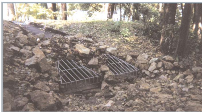
Riprap provides energy dissipation of storm water at outlets, thus reducing erosion potential.
