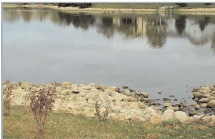
Detention ponds temporarily store and treat storm water until it is discharged.
