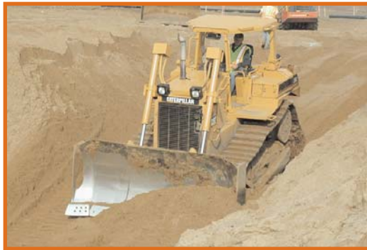
Sediment control during construction will prevent off-site damage.
