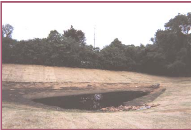
Erosion control blanket was successfully used on the upper slopes to reduce erosion into the pond.
