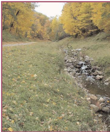
A swale with field stone was used to direct water and reduce erosion from this site.
