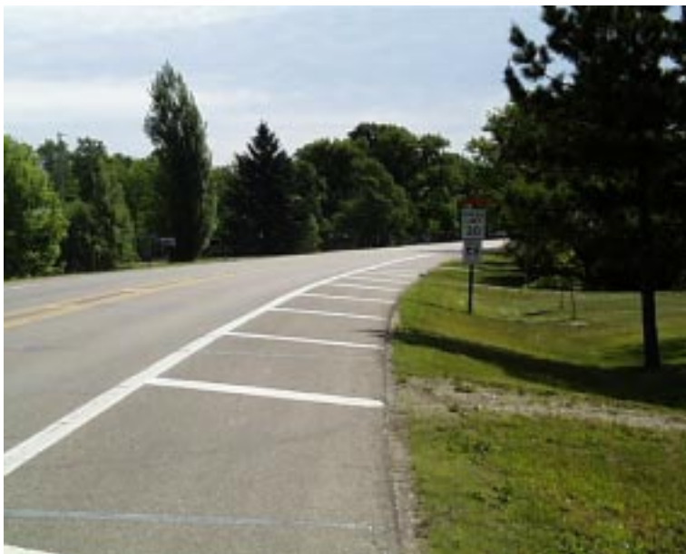
Figure 3.3 Shoulder Stripes—Twin Lakes
