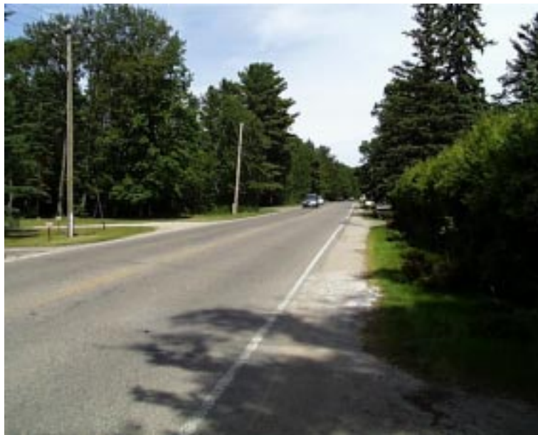
Figure 3.4 Unpaved Shoulders—Bemidji
