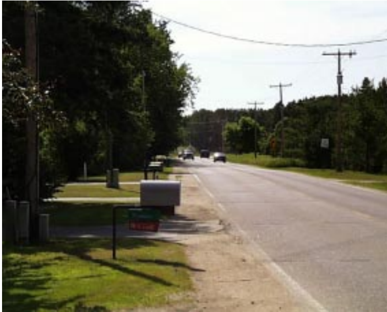
Figure 3.5 Narrow Shoulders—Bemidji
