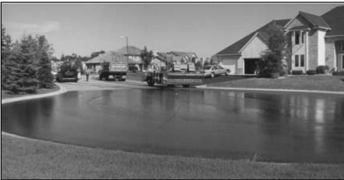
Figure 7.8. Wrong way to sealcoat a cul-de-sac (emulsion will “break” before chips are placed and rolled)
