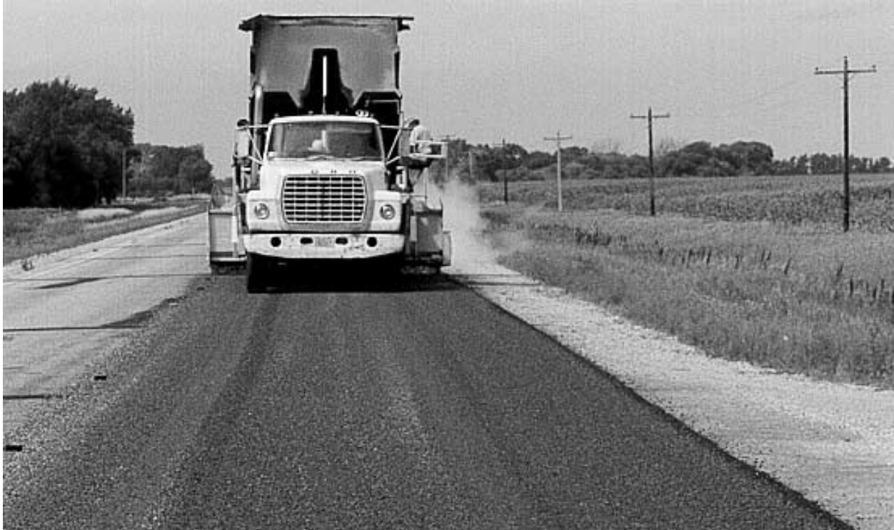
Figure 5.4. Darker wheel paths indicate binder has risen near the top of the aggregate.
