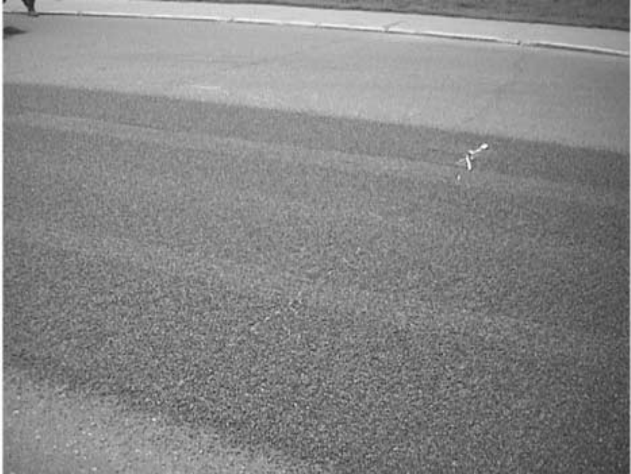
Figure 6.2. The rubber mats are covered with aggregate from the chip spreader
