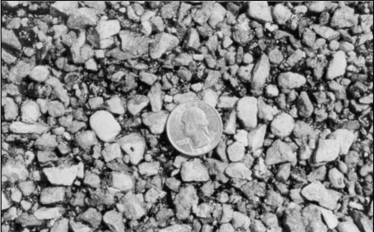
Figure 5.2. Not enough binder (binder is too low)
