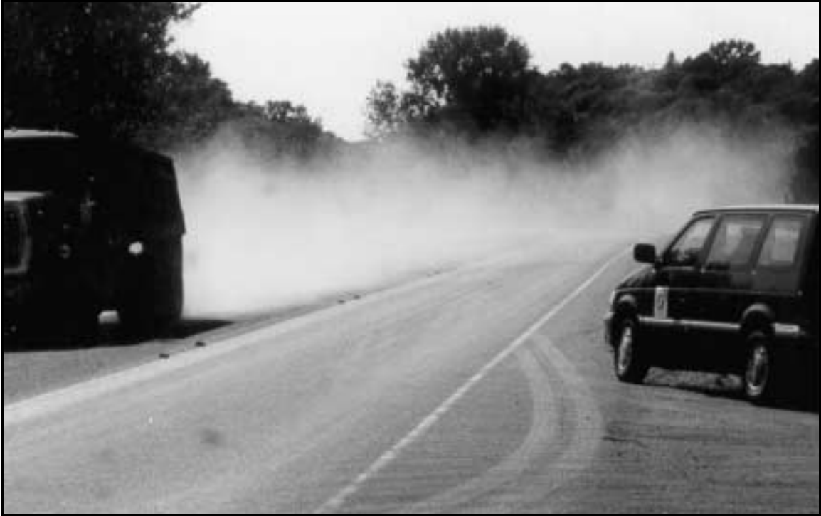
Figure 2.7. Evidence of a dusty aggregate
