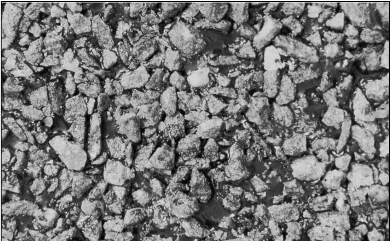
Figure 5.3. Correct amount of binder (binder has risen to top of chips)
