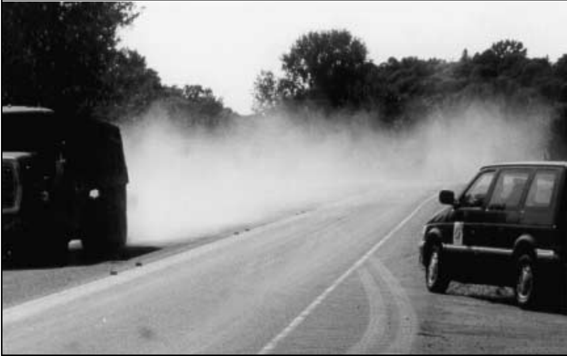
Figure 7.6. Evidence of a dusty aggregate
