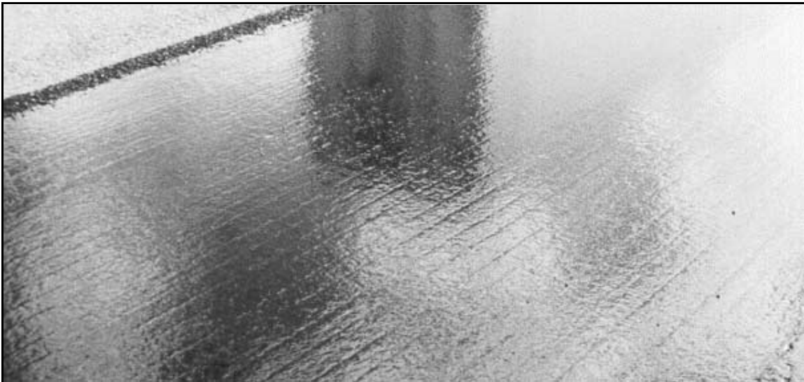
Figure 7.1. Example of streaking caused by incorrect spray bar height (notice streaks)
