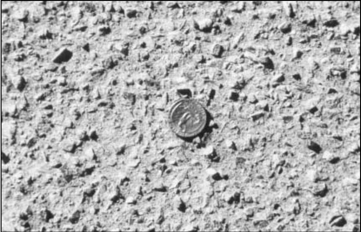
Figure 2.9. Dusty aggregate after sweeping (notice most of the large aggregate is missing)
