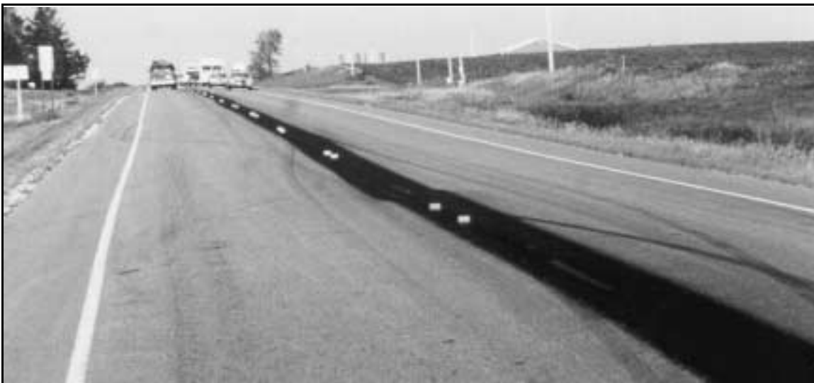
Figure 7.7. Fog seal on centerline prior to seal coat to prevent excess absorption
